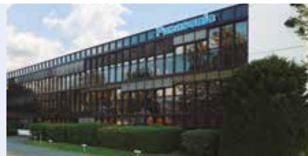
Panasonic Marketing Europe GmbH - Panasonic Air Conditioning in Wiesbaden, Germania.
